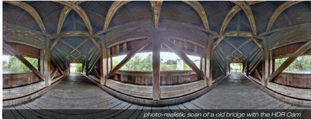
photo-realistic scan of a old bridge with the HDR Cam
